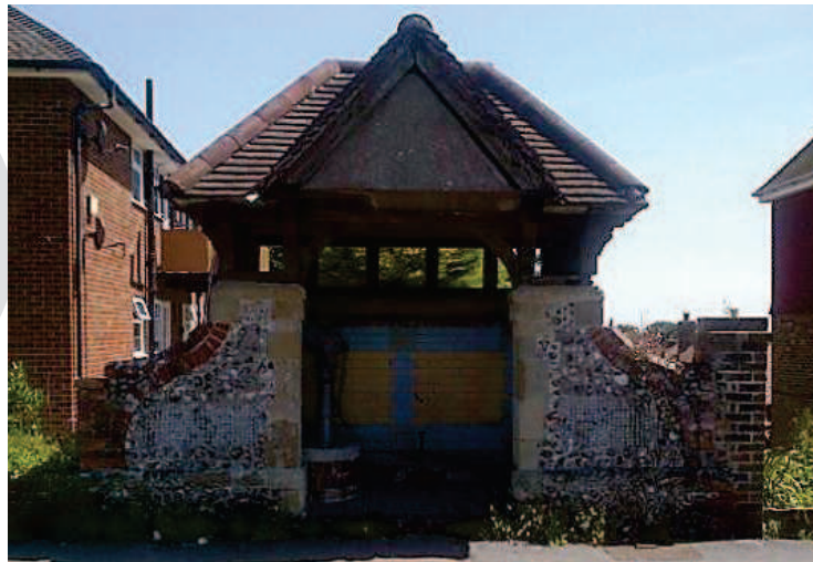
Willingdon Village Pump House (An existing locally listed building)
